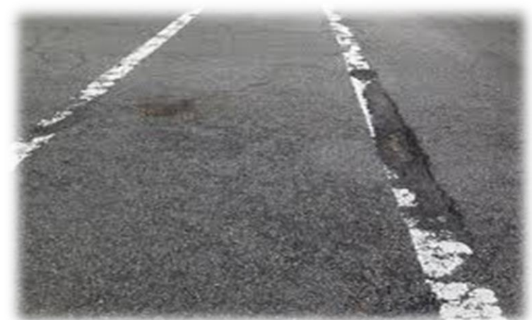
Faded road markings with wear index > 20
